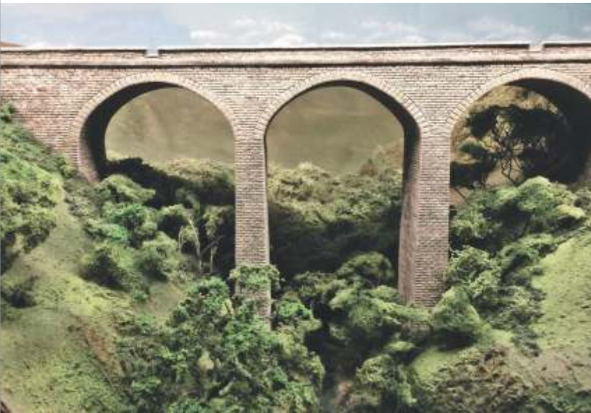
A high arched bridge spanning a gorge
