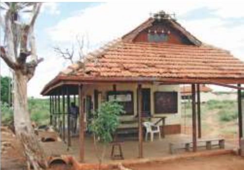
Kiosk-size station at Tsavo
