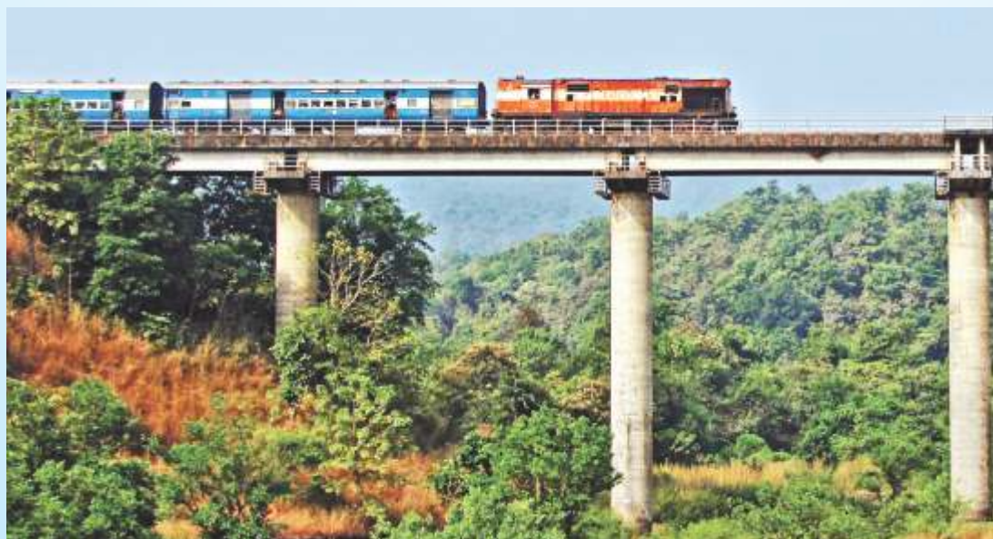
Romance of the railway: a train glides across a viaduct
