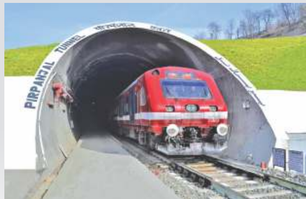
Entry to Pir Panjal tunnel
