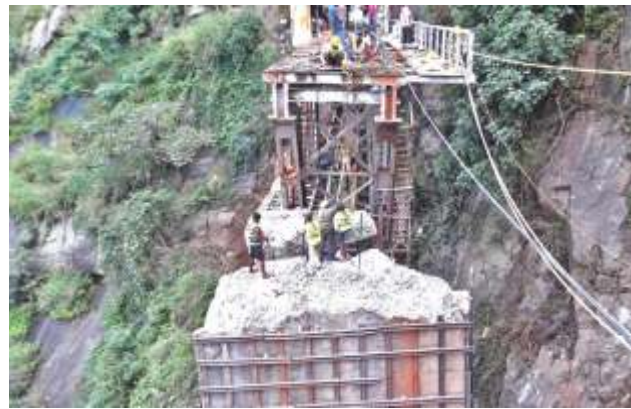
Working on the damaged bridge
