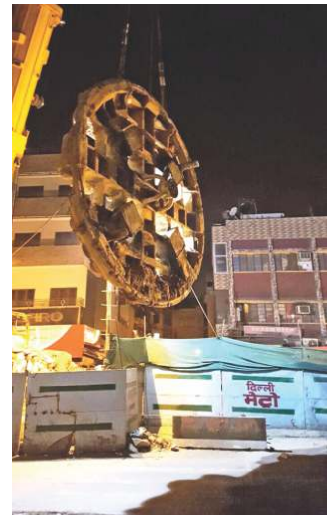
The TBM's cutter
