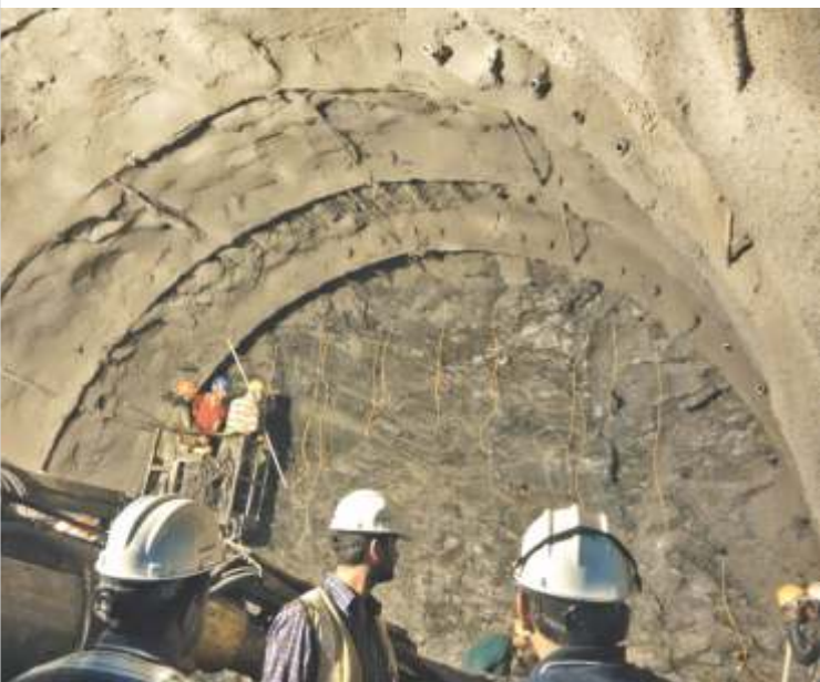
Tunnel T48. Loading and charging
