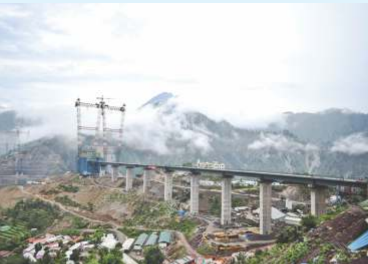
A view of the viaduct of the Chenab bridge
