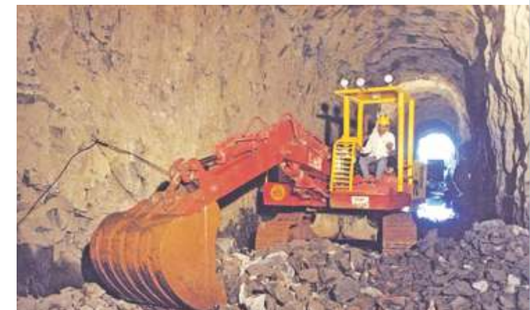
An excavator at work inside a tunnel
