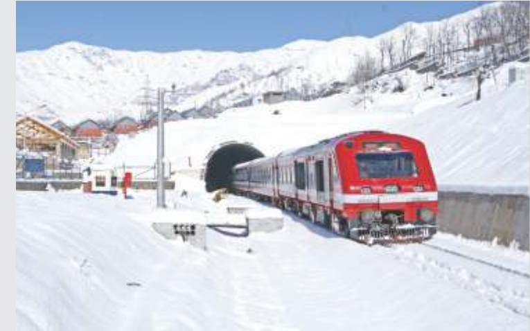
Pir Panjal Tunnel in winter
