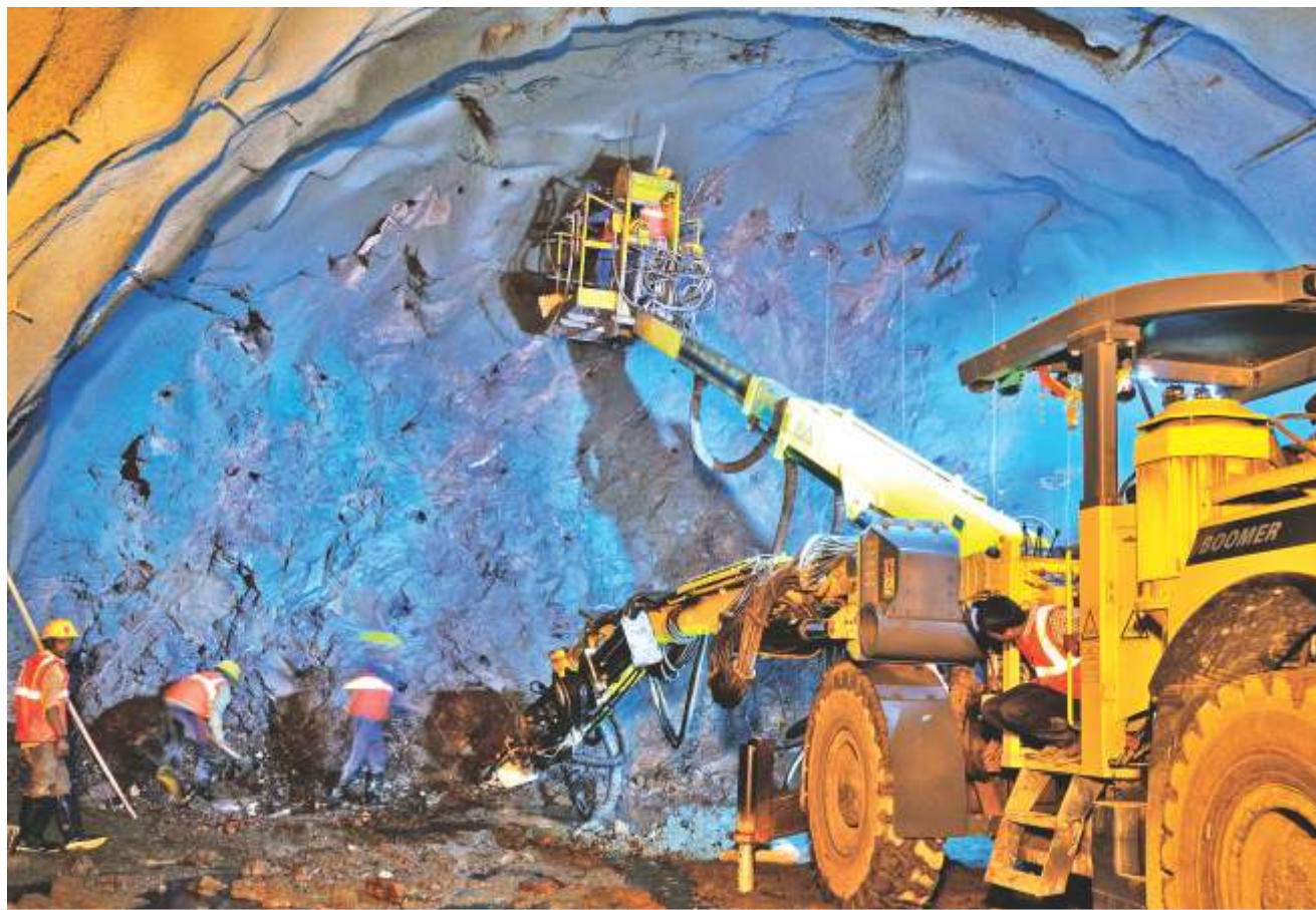
Loading and charging of explosives in Tunnel T13
