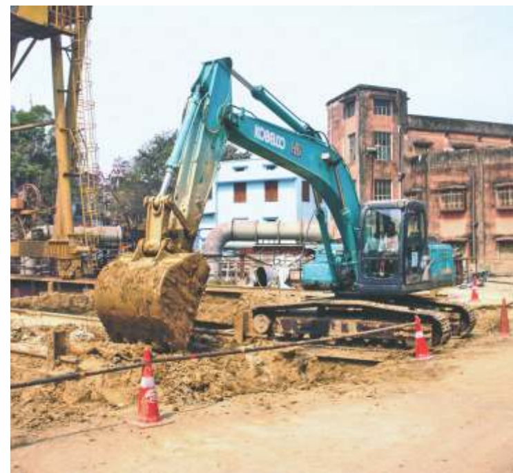
Earth mover that loads excavated debris into road vehicles
