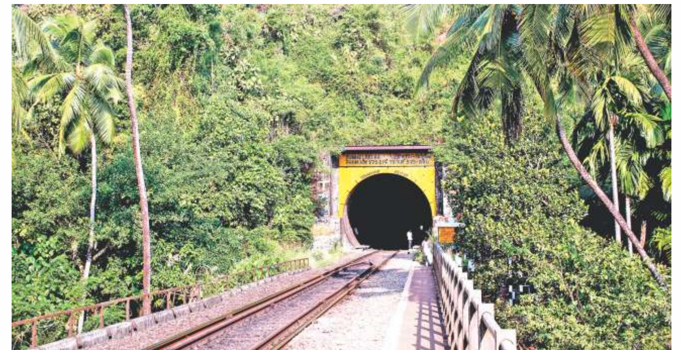
Completed South face portal of shield tunnel at Honnavar
