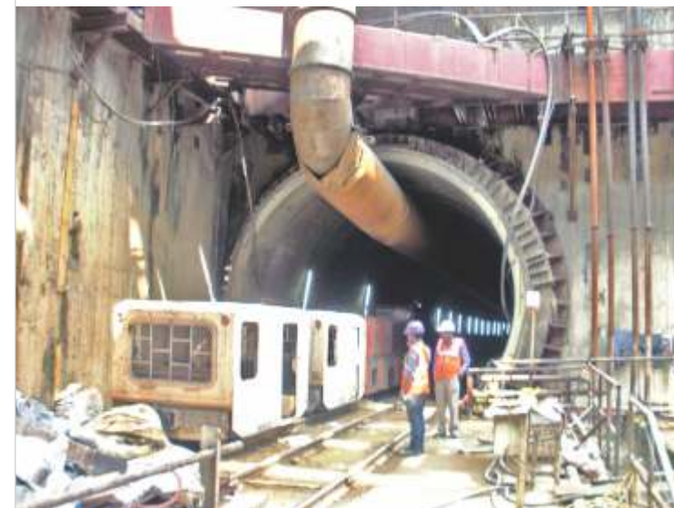
Entry to tunnel
