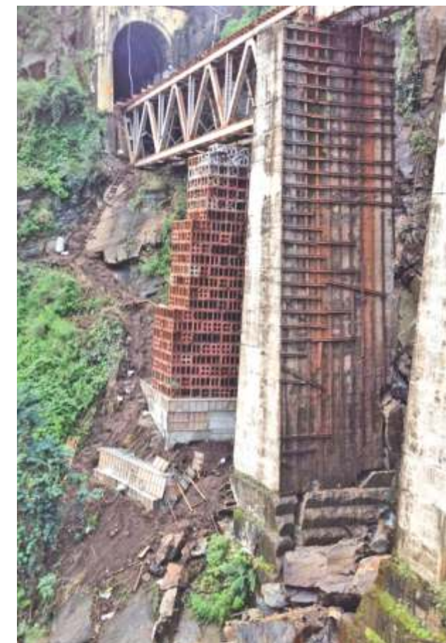
Temporary support ready
