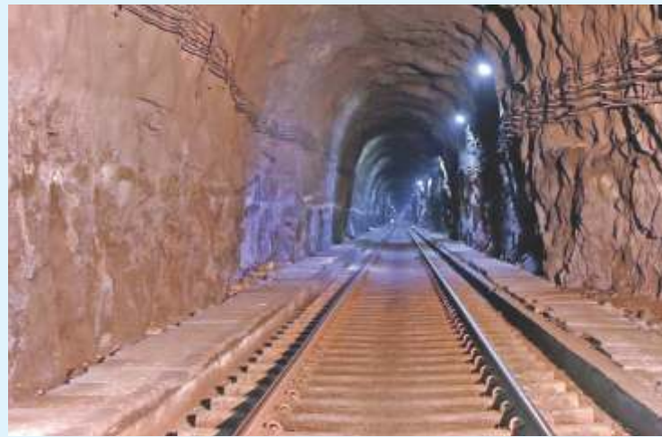
Ballast-less track in Karbude tunnel of Konkan Railway
