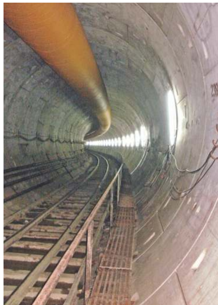
Inside the tunnel. Note the walkway along the right
