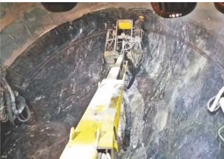
Tunnel T48. Wire mesh fixing
