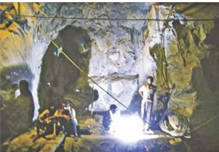
Work in progress in a hard rock tunnel
