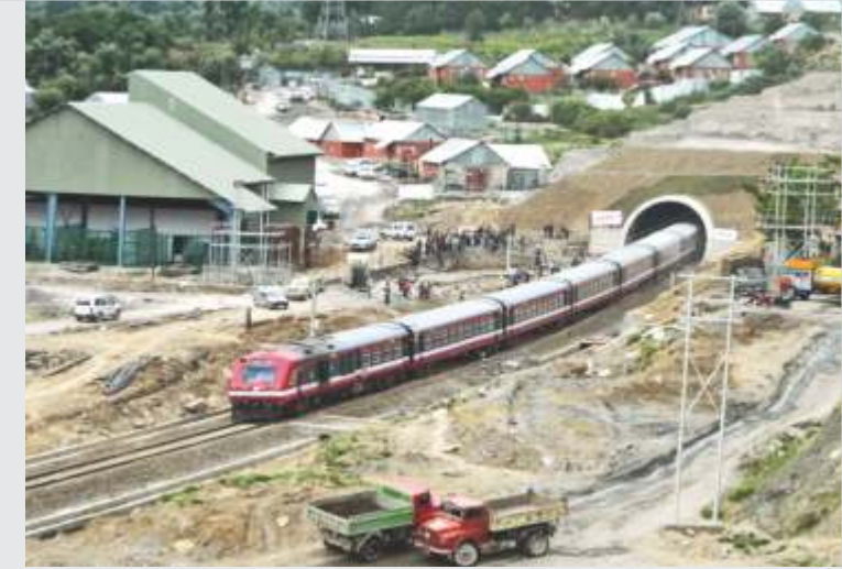
Train emerging from Pir Panjal Tunnel
