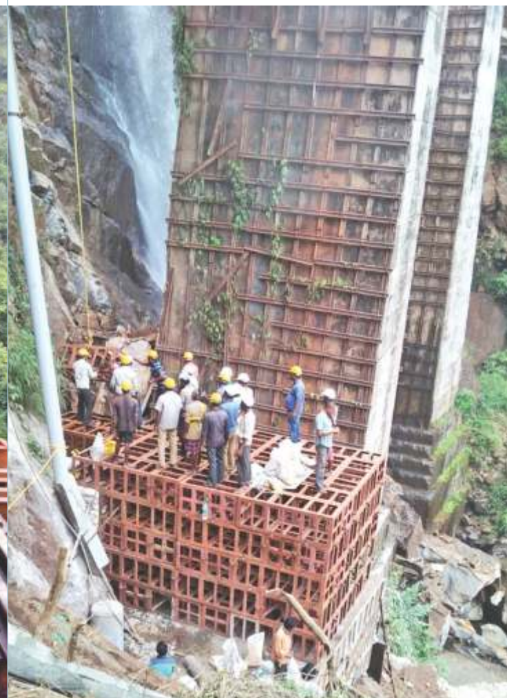
Building of the crib support
