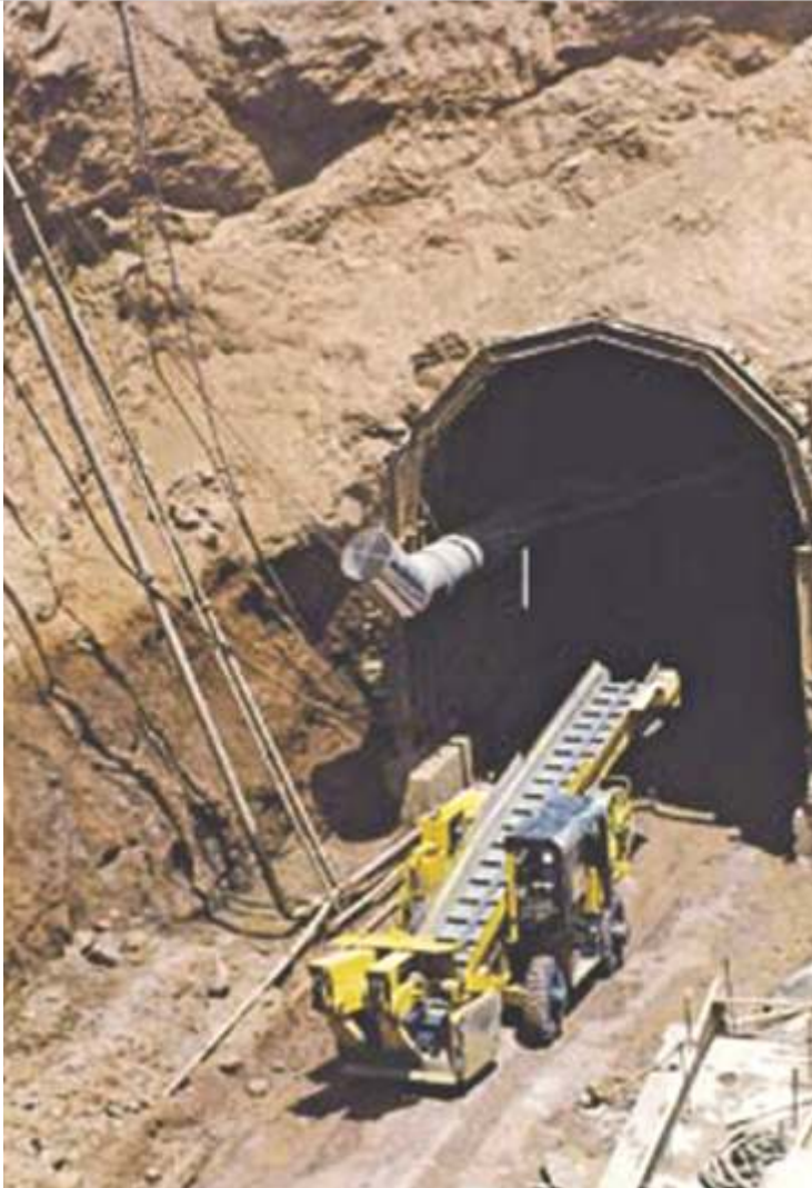
Hagglund loader moving into a tunnel
