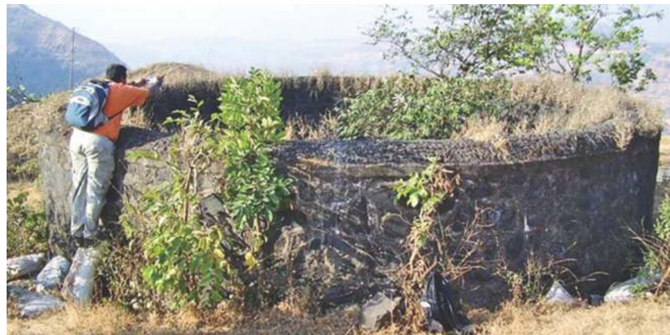
Wall built around ventilation shaft of Tunnel No. 49
