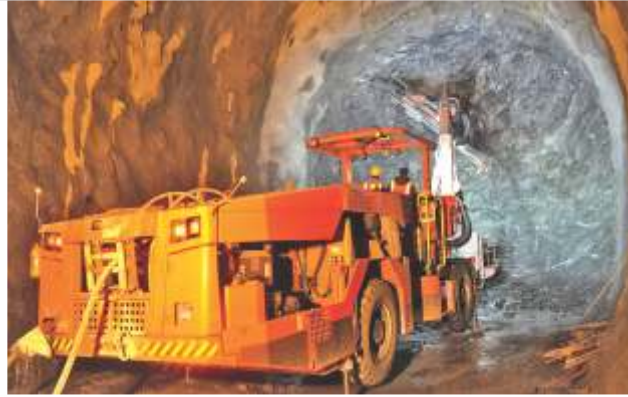
A boomer in escape Tunnel T48
