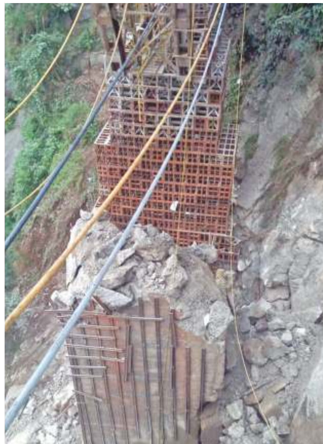
Partly dismantled pier
