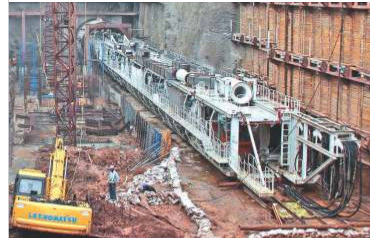
A Tunnel Boring Machine (TBM)
