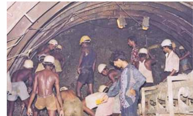
Heading work in progress
