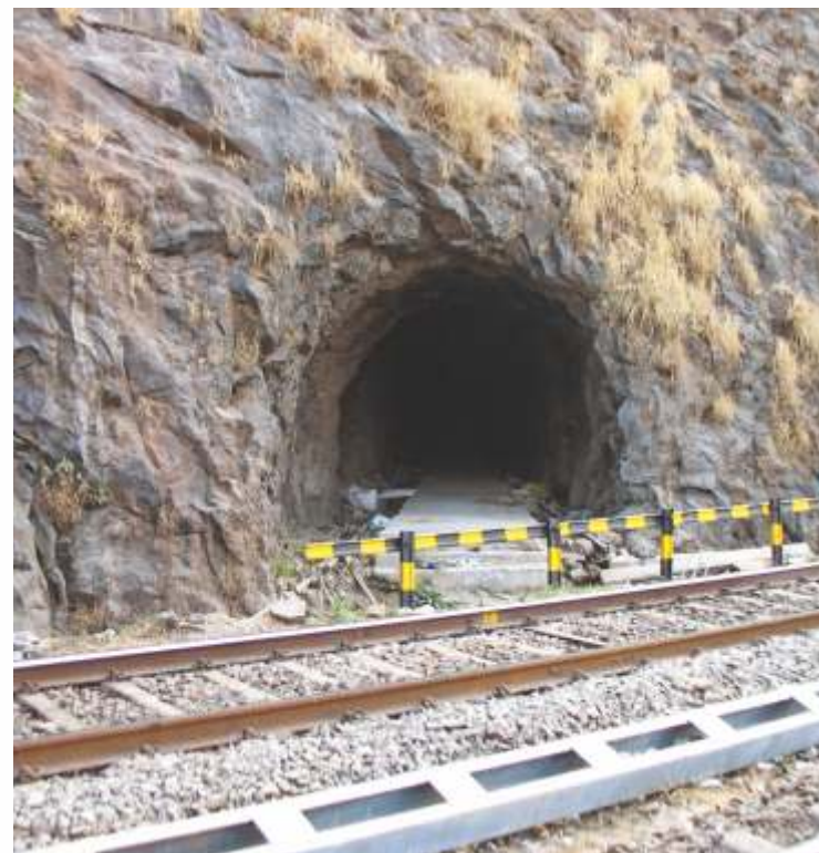
Portal of service tunnel
