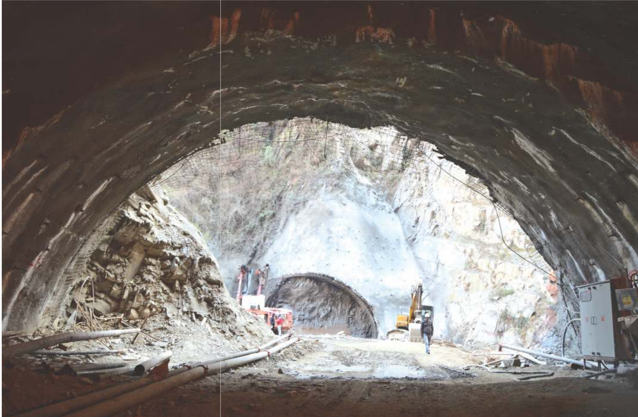
Portal development work on Tunnel T49
