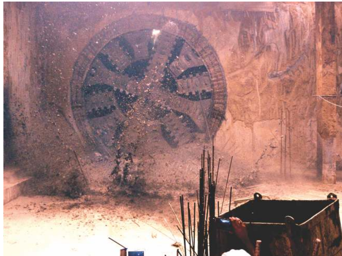
Breaking through the end of the tunnel at the Red Fort
