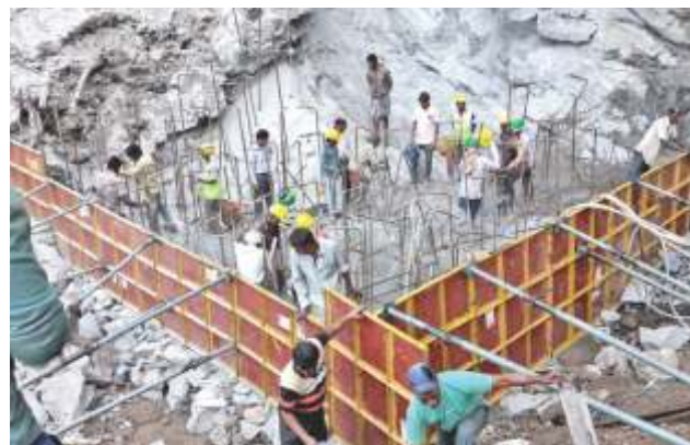
Building of the new pier
