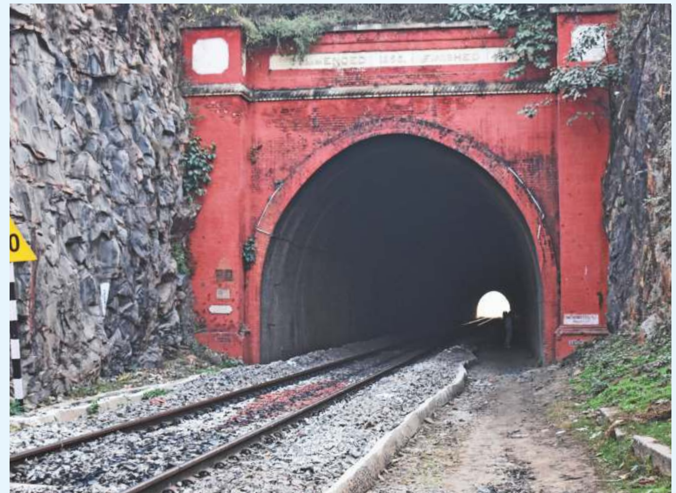
Western end of the Jamalpur tunnel
