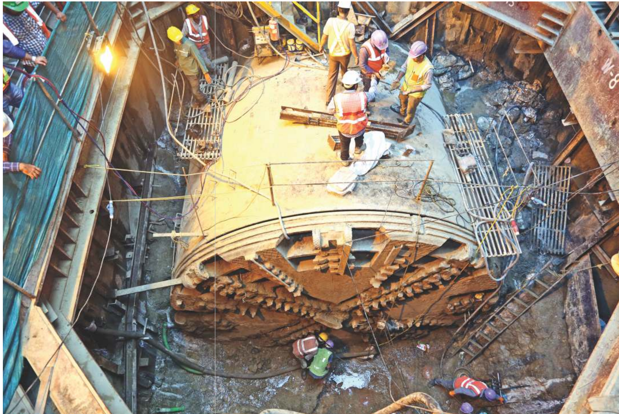
Retrieval of the TBM at the Rameshwar Nagar Gurudwara shaft
