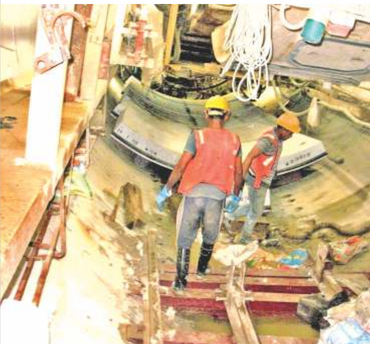
Pre-cast concrete sections lining the tunnel
