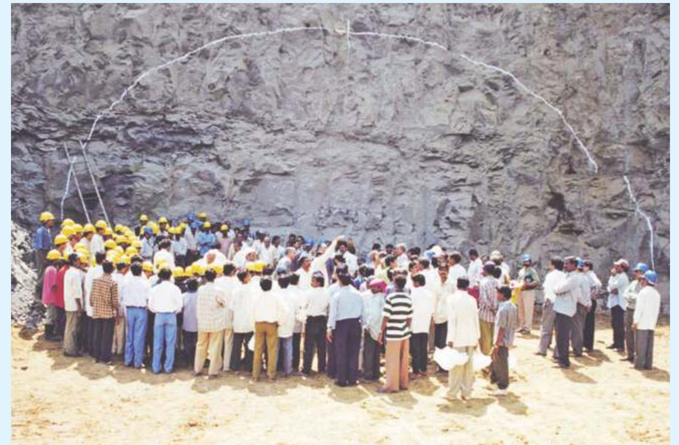
Profile marking for initial blast
