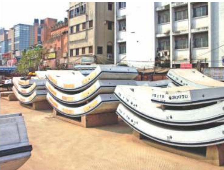
Sets of pre-cast concrete sections used for lining the tunnel
