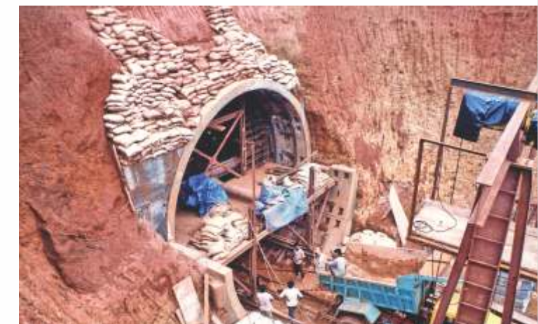
Benching work being undertaken
