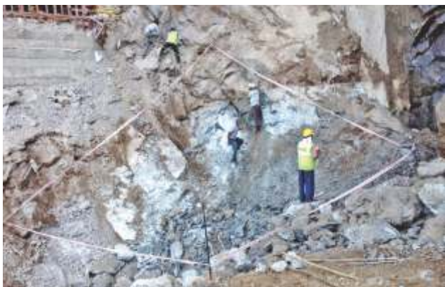
Marking of the foundation of the new pier
