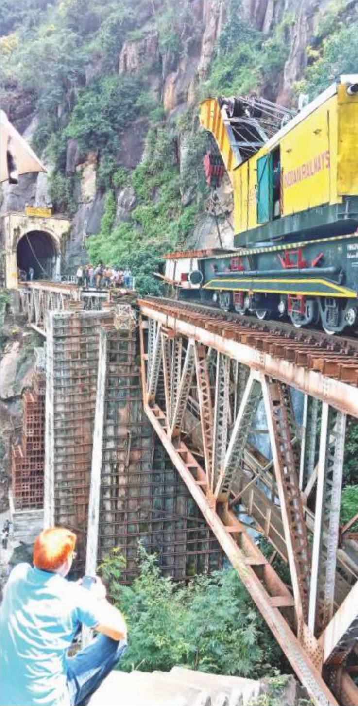
The 120-T crane working on the central short girder
