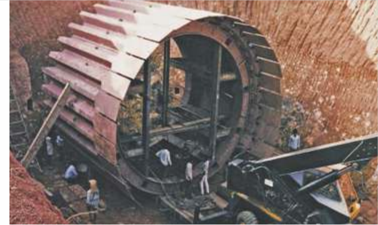
Shield tunnelling blades being assembled
