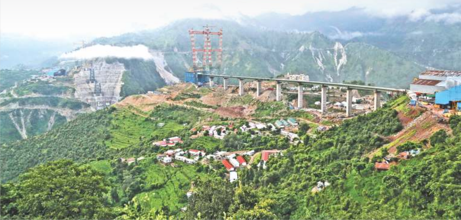
Panoramic view of Chenab viaduct
