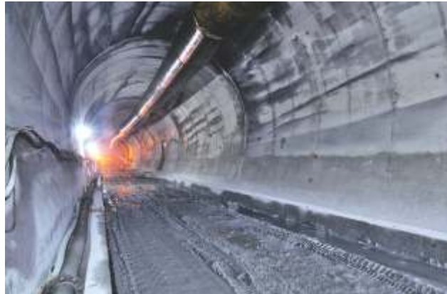
View of Tunnel T49 after lining
