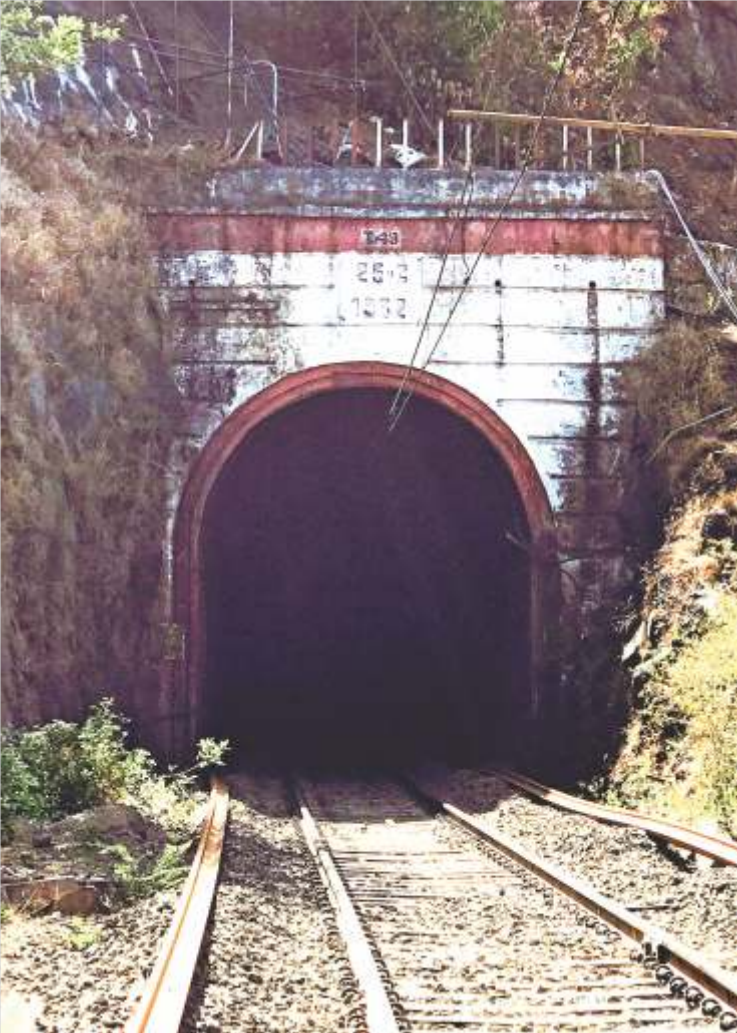
Tunnel No 49 (25C) with year of construction
