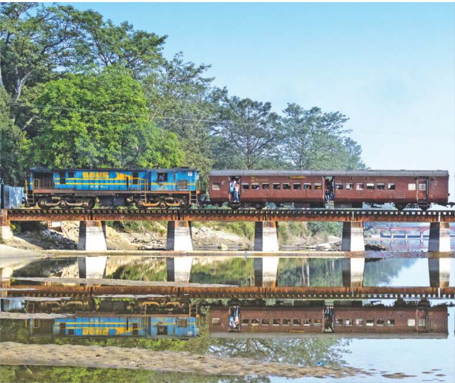
The Terai is irrigated by a large number of rivers and canals. The first train of the day crosses one such canal near Pilibhit
