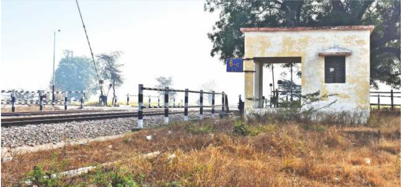
Manned level crossing with locked cabin
