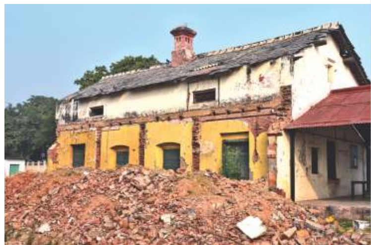
Demolished portion of station building
