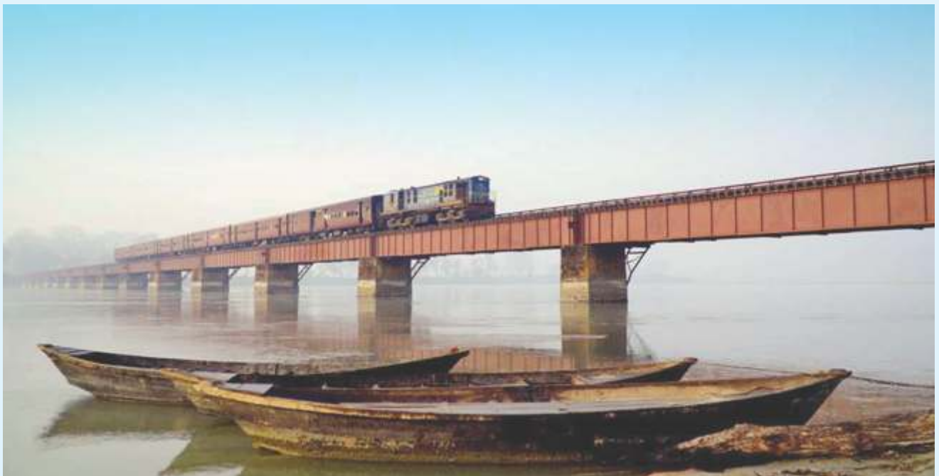
Train crossing bridge over the Sharda River near Palia Kalan
