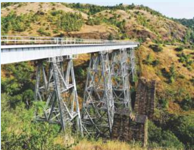
Ravine viaduct No. 2 on Patalpani-Kalakund section
