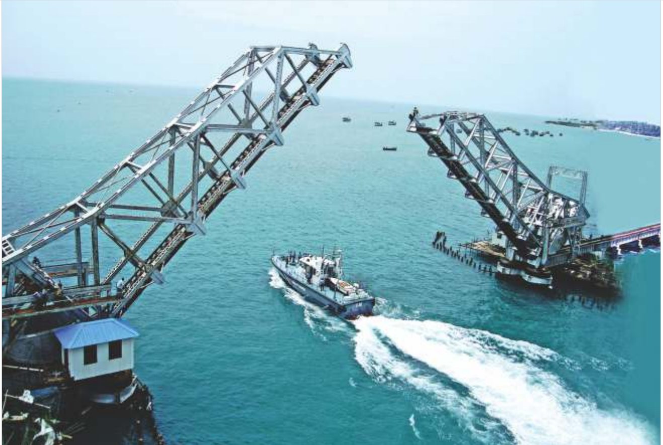
Spans of the bridge lift for a ship to pass
