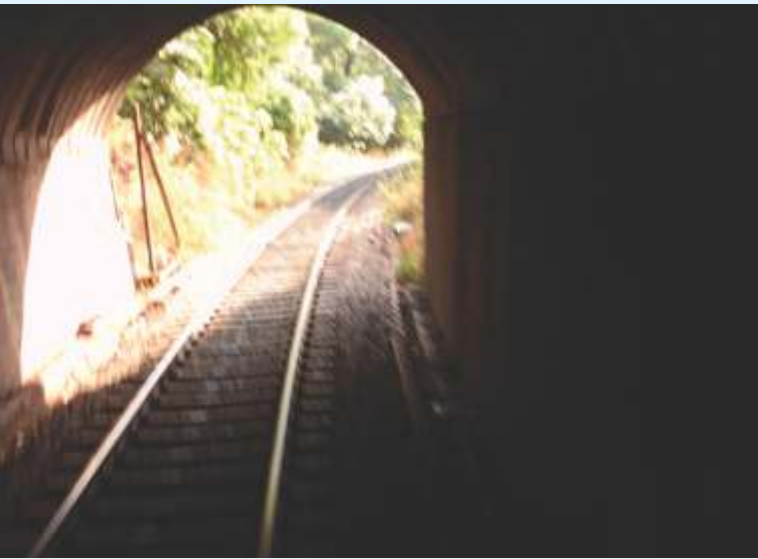
The exit from tunnel No.2
