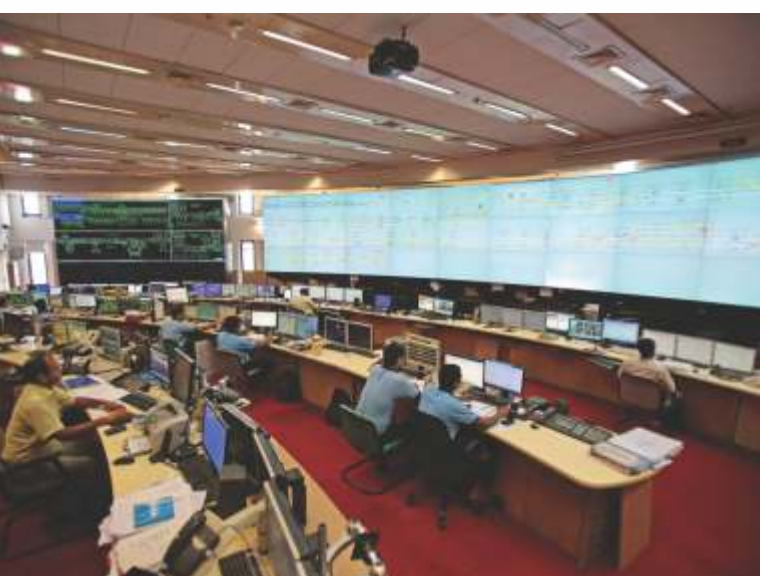
In the Control Room
