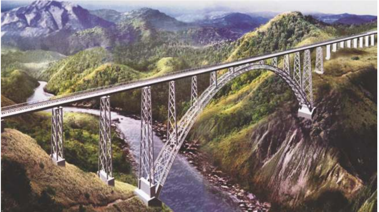
Artist's impression of the bridge across the Chenab. When ready, this will be the highest bridge of its type in the world
