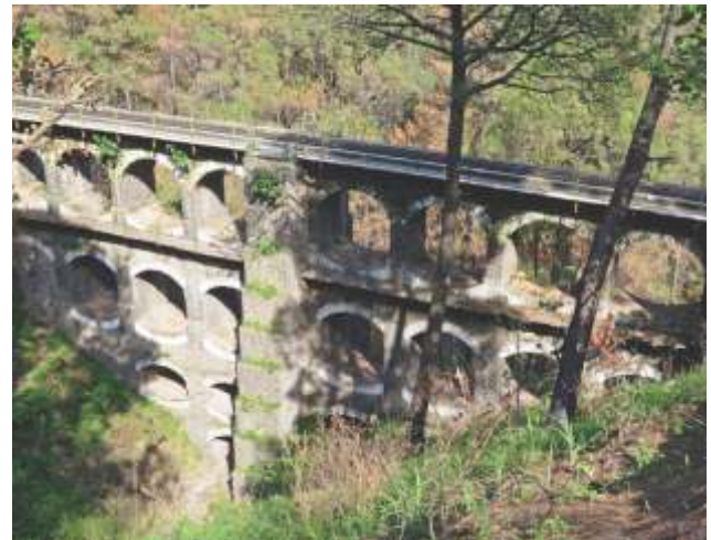
Multi-tiered arch bridge on the Kalka-Shimla Railway
