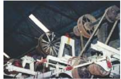
Driven overhead line shaft
