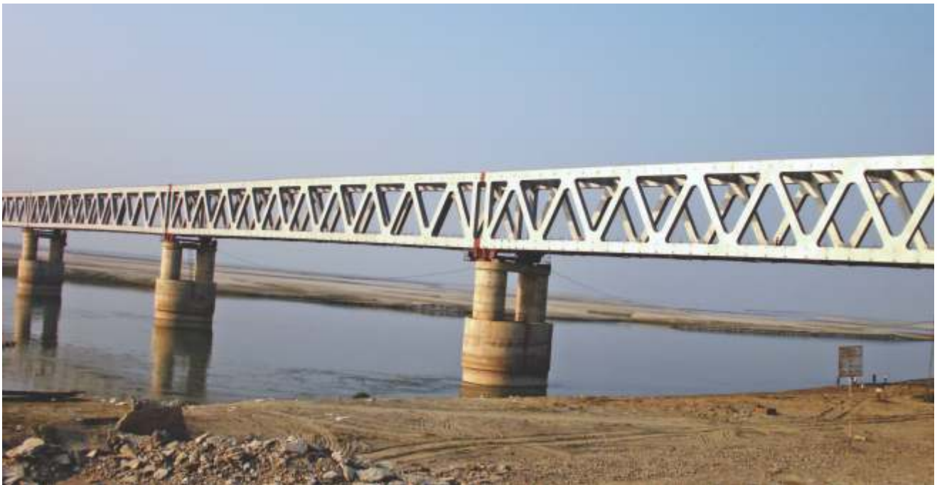
Bhogibeel bridge with girders
