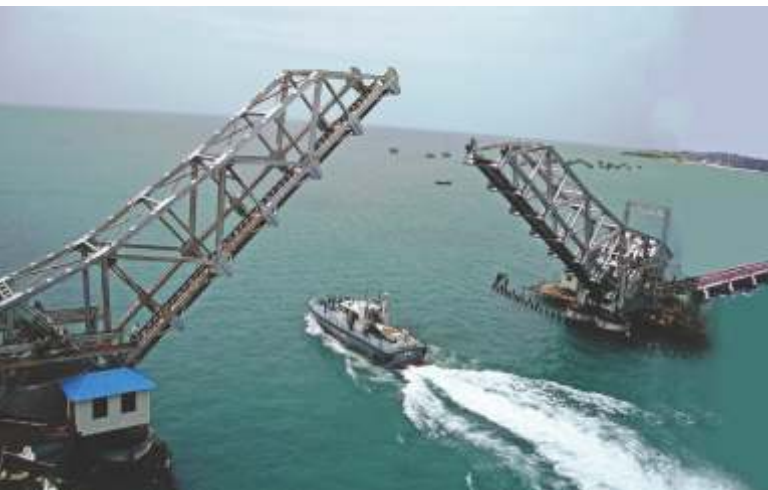
Pamban bridge - open to ship movement
