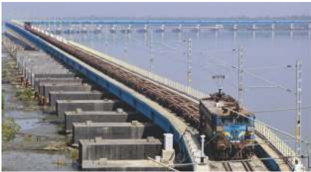
Vallarpadam Bridge at Kochi, currently the longest bridge in India
