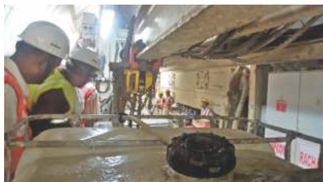
Inside the tunnel
