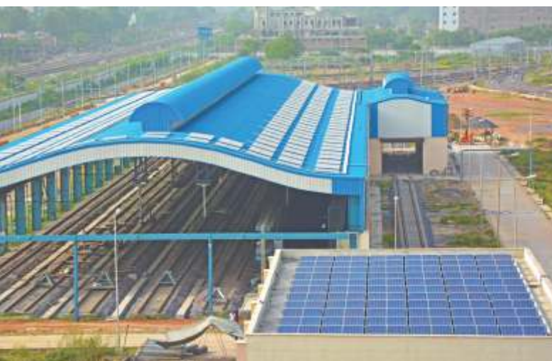
Metro repair facility. Note the solar panels on the roof
