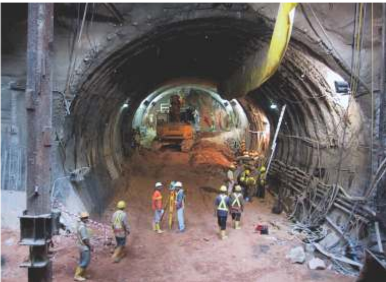
Construction in progress. Note the mandatory wearing of safety helmets, etc.
