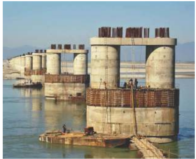
Bhogibeel Bridge - Work in progress on the piers
