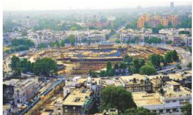
Bird's-eye view of the Connaught Place Central Park during renovation
