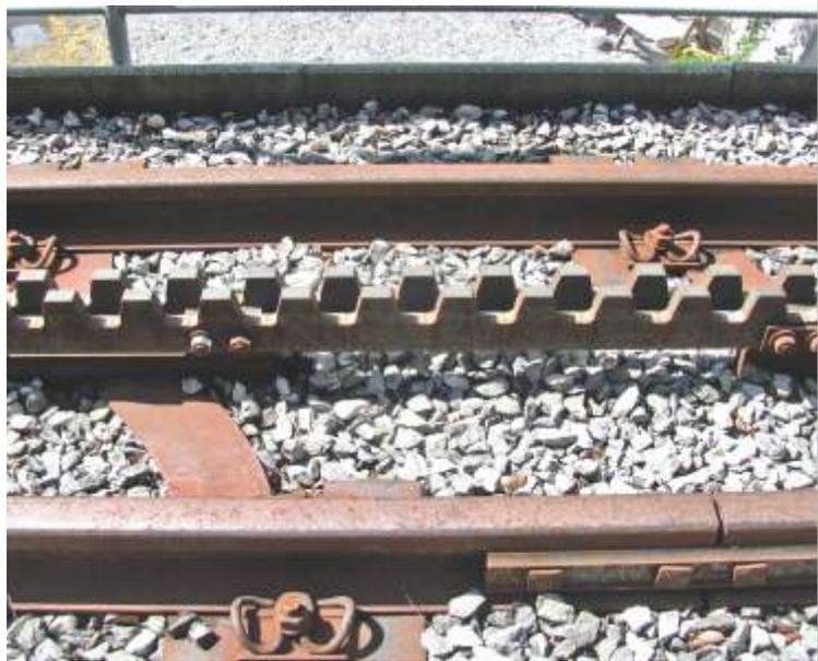
BRB utilizes Abt dual rack and pinion system on the entire stretch
