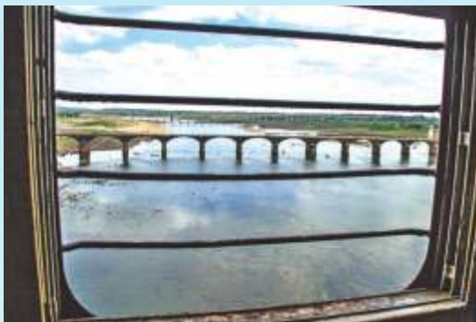
▲ From the window of a train on the Omkareshwar bridge
