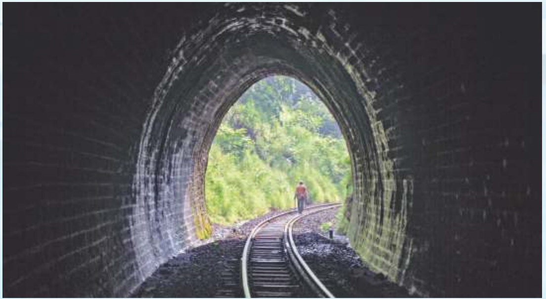
▲ Gangman inspecting track inside a tunnel
