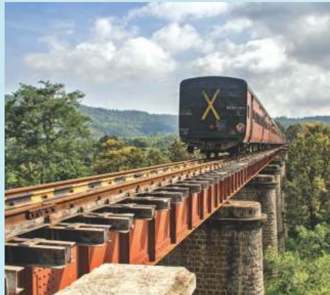
▲ Passenger train crossing the Dhulghat spiral
