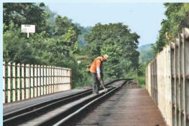
▲ A gangman inspects the line on Ravine viaduct No. 1
