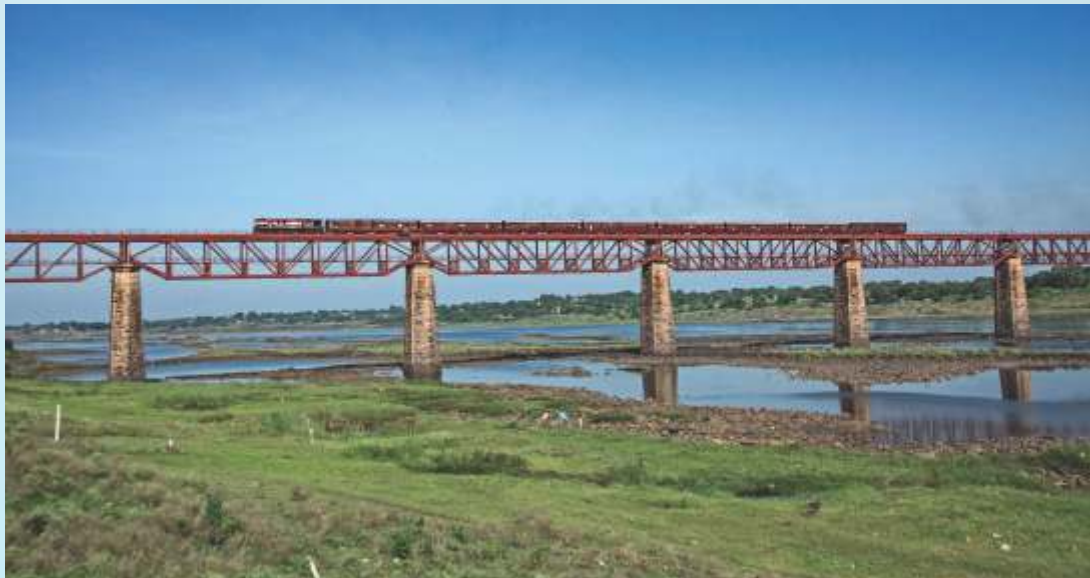
▲ Train 52988 on the Omkareshwar bridge
