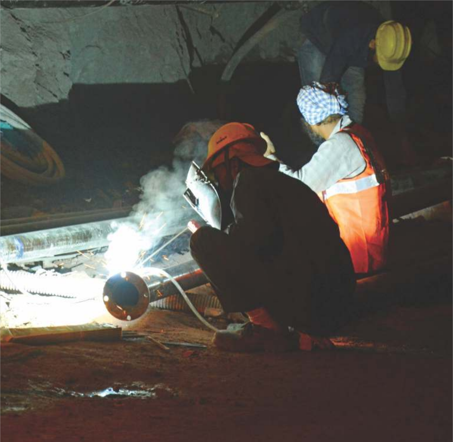
Welders at work inside the tunnel
