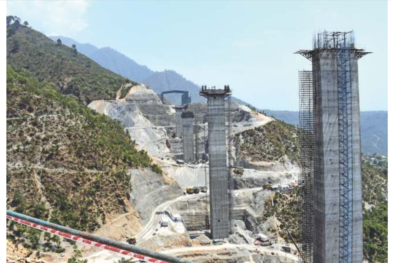
View of Bridge No. 39 from the Banihal end
