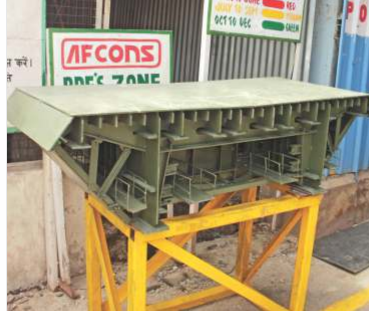
A model of one of the steel segments of the viaduct
