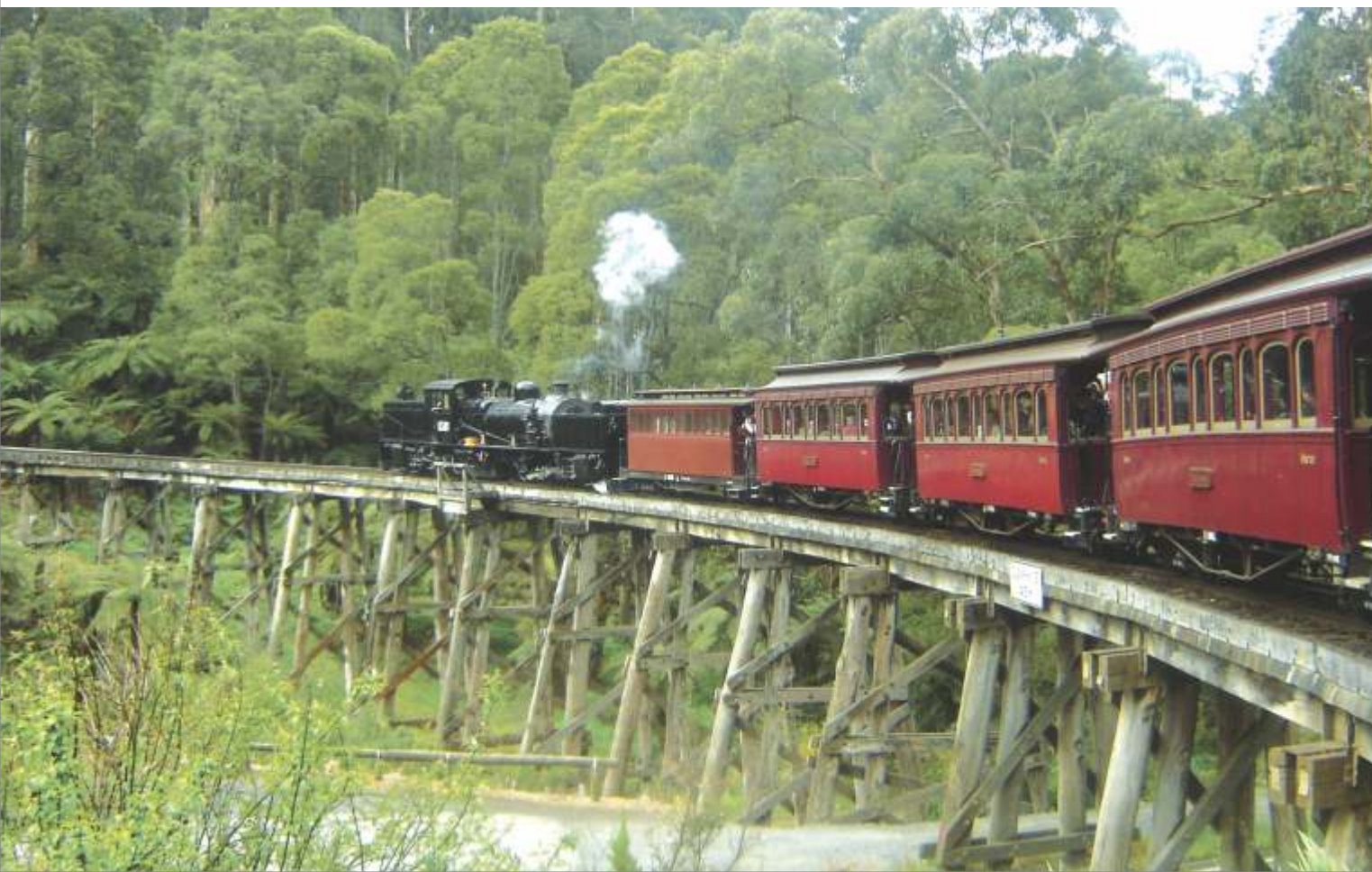
Puffing over a trestle bridge
