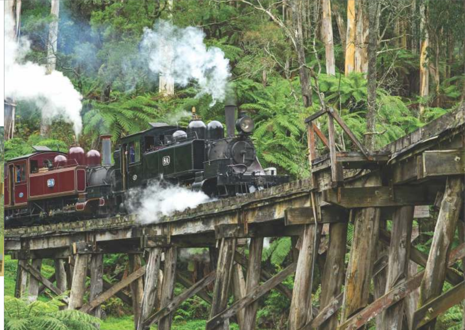
Puffing Billy passing over the Monbulk Creek trestle bridge
