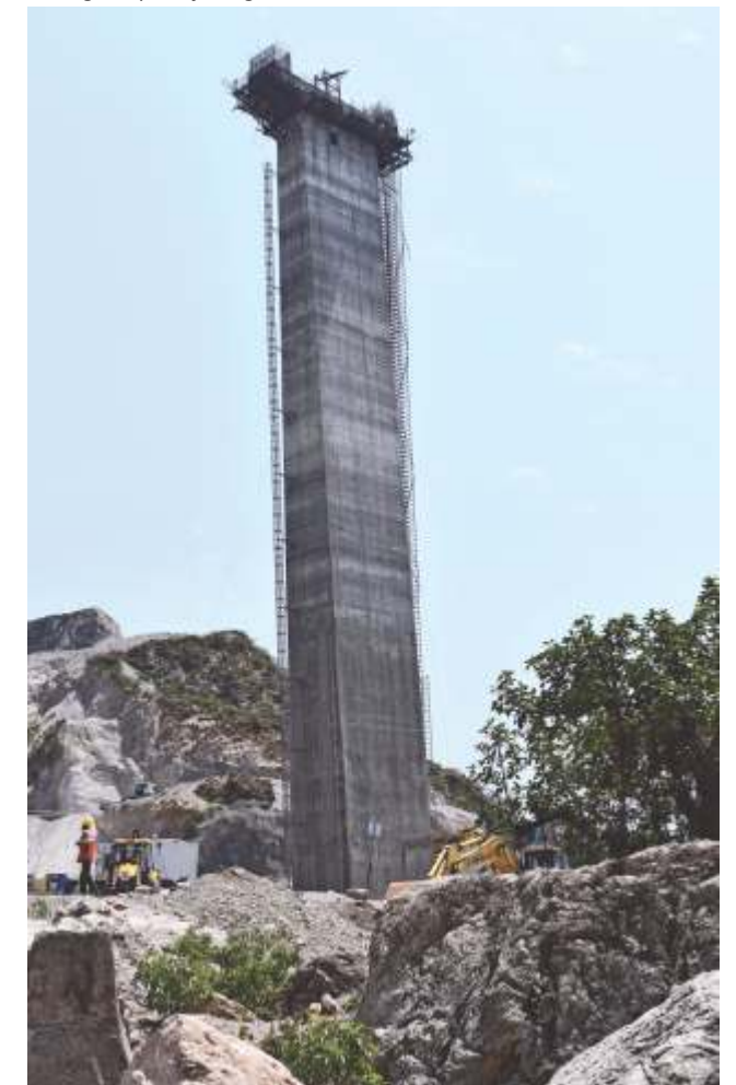
The highest pier of Bridge No. 39
