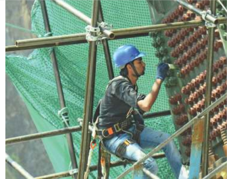
Applying protective paint
