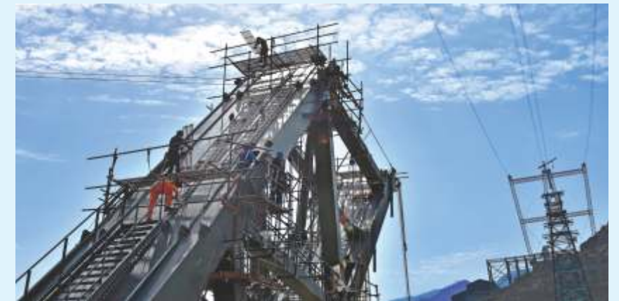
Steel arch of the Chenab bridge under construction
