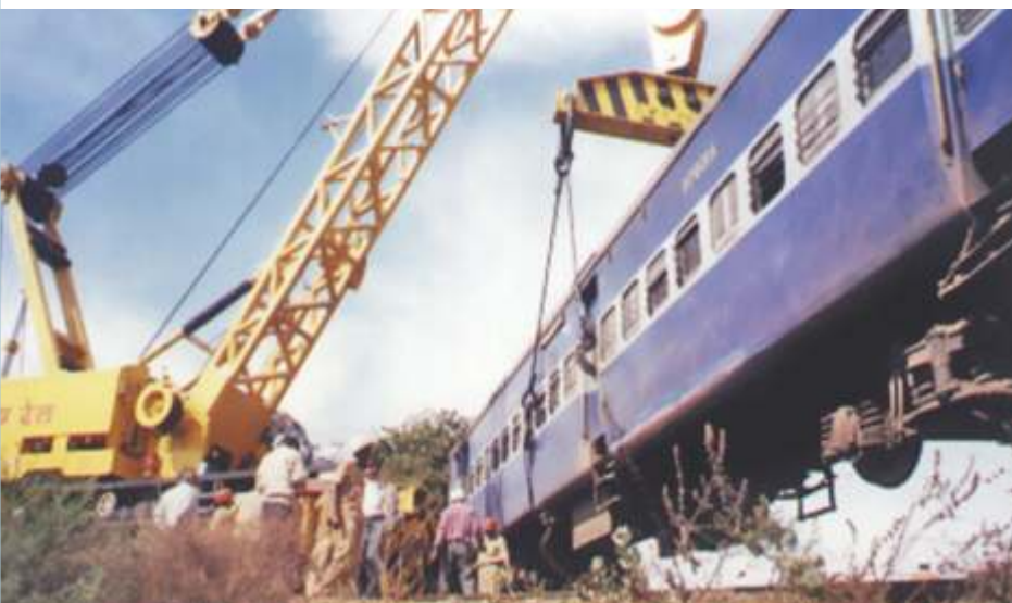
At an accident site – the crane in action
