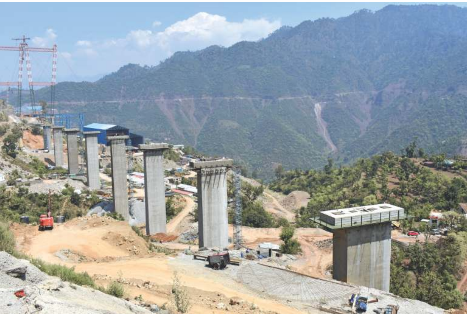
Closer look at the piers of Bridge No. 43
