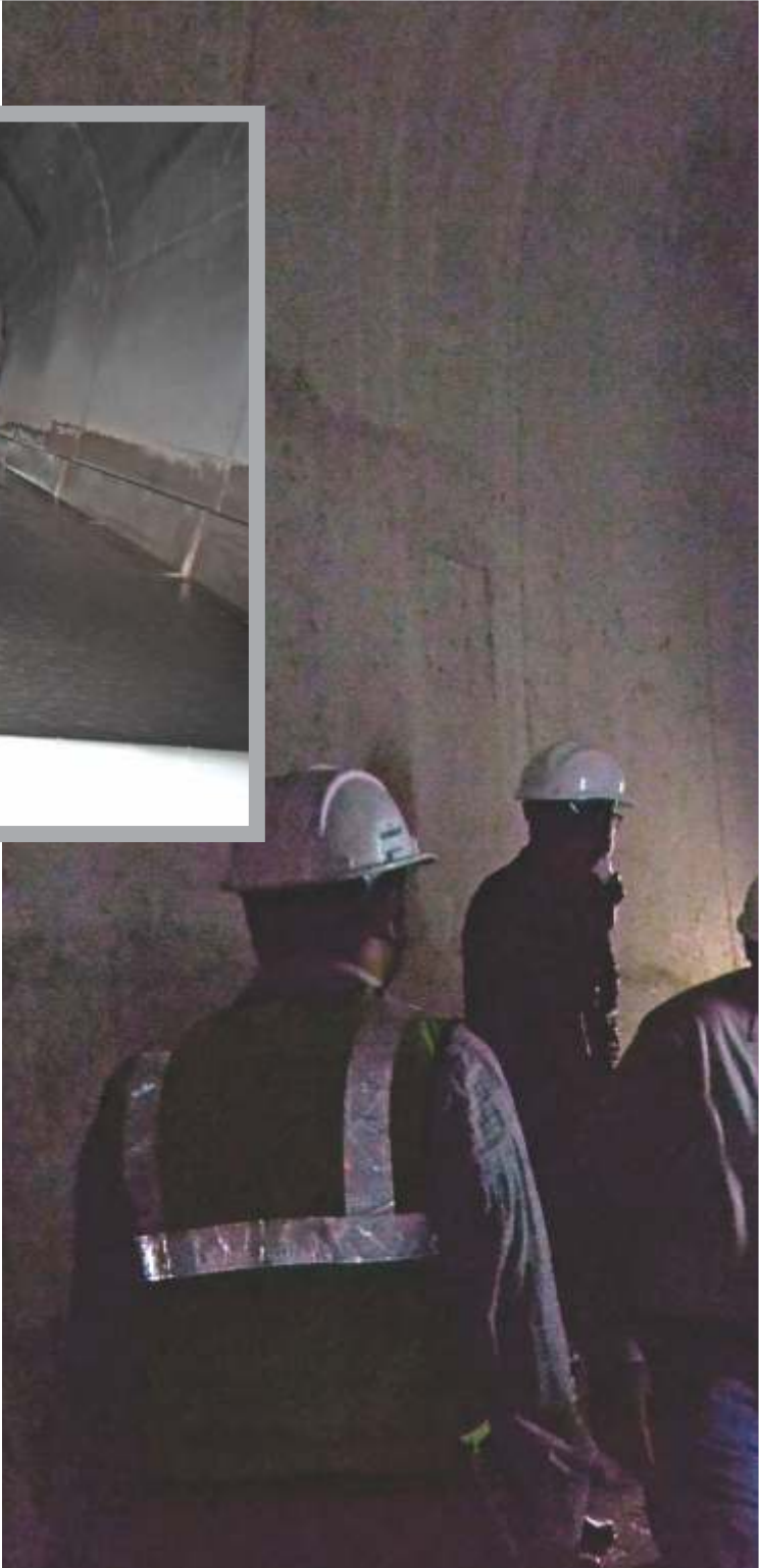
Inside Tunnel No. 5
