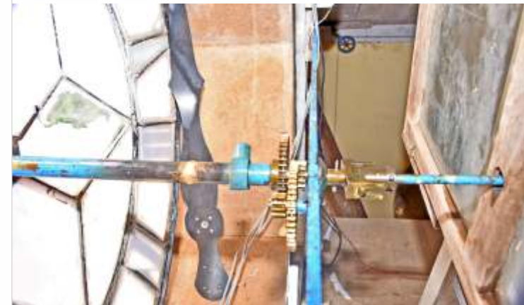
Some of the gears and components that were repaired
