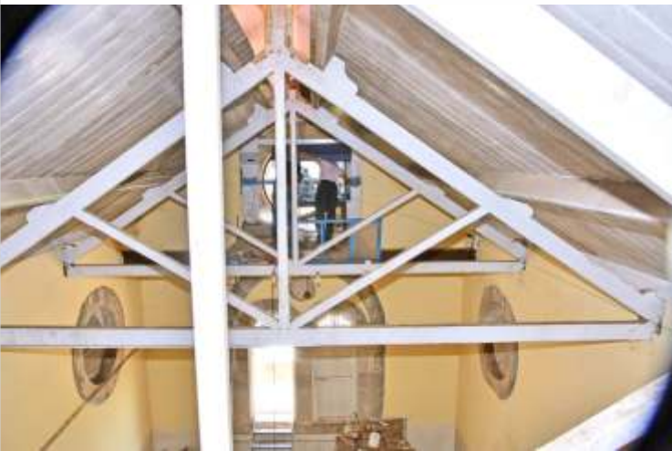
Location of the clock above the first floor
