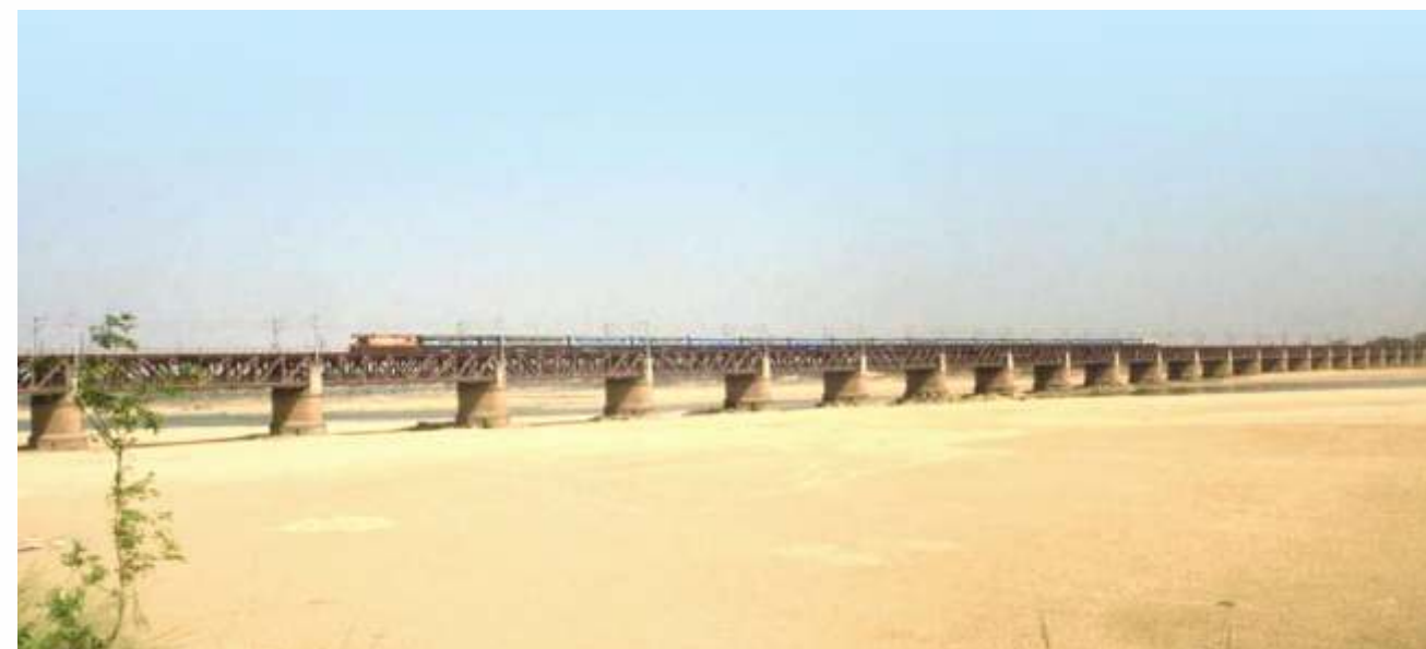
Bridge across the Sone River near Arrah in Bihar. The was the first major railway bridge built in India. Simms' advise on the building of this bridge ensured its construction
