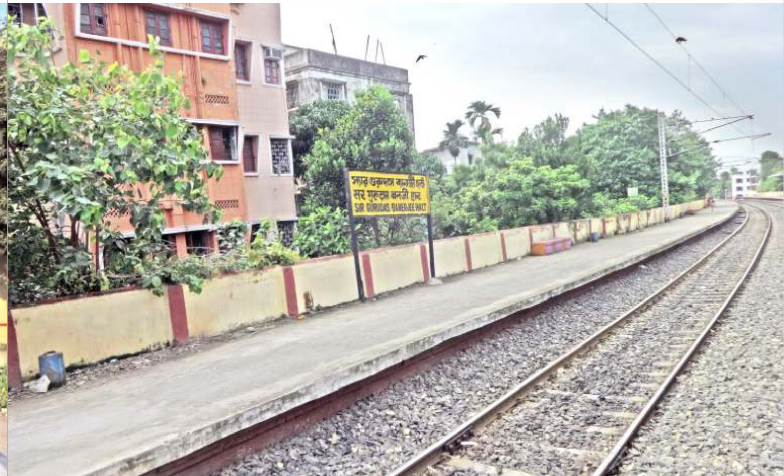
Sir Gurus Das Banerjee Halt, the station set up to bypass Sealdah terminus Dum Dum Junction – where you connect with three other lines
