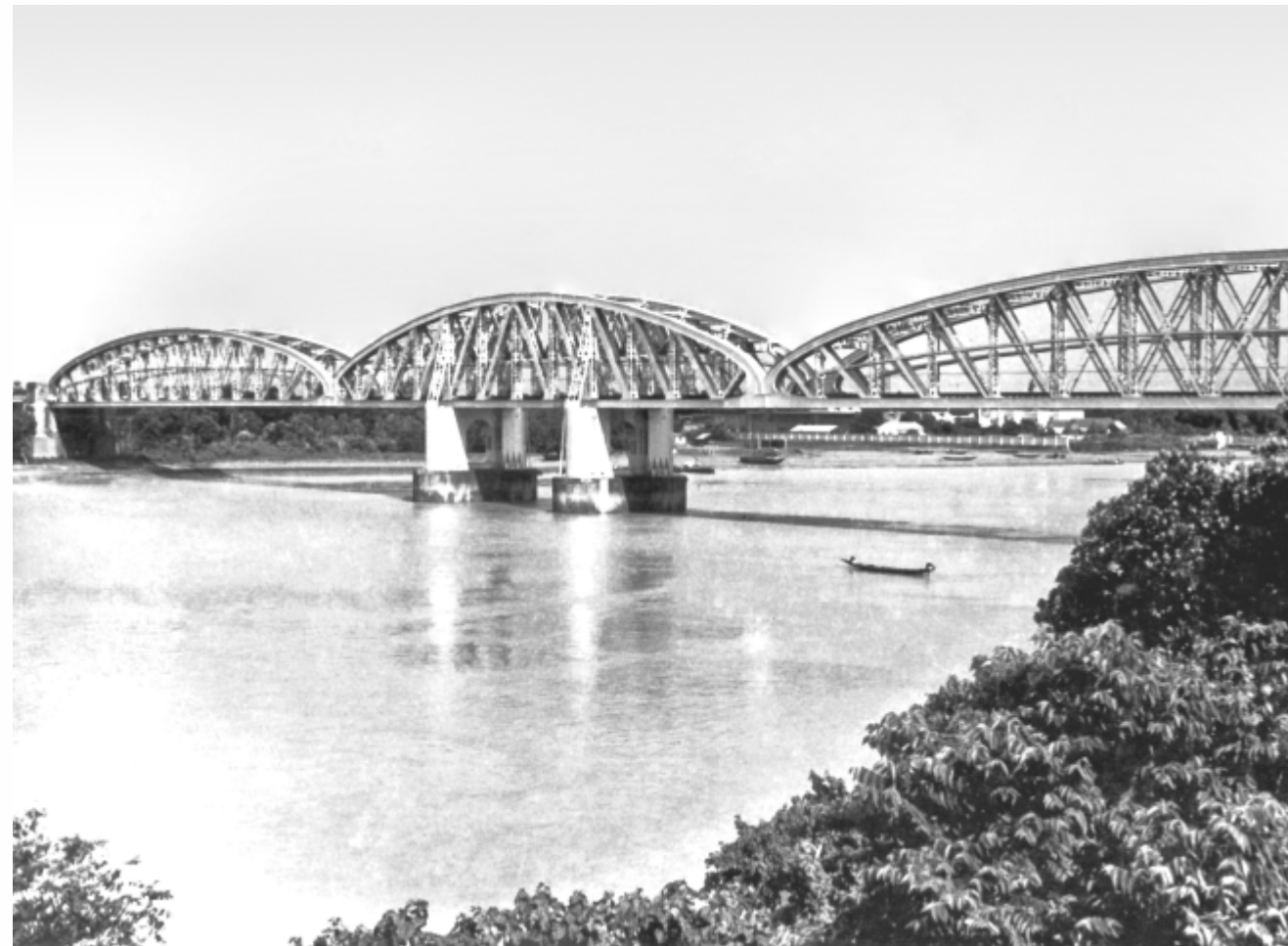
1887-commissioned erstwhile Jubilee bridge was built to double line requirements
