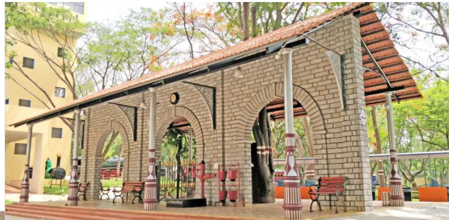
All in vintage style: The tiled roof, the ornate pillars, the weighing machine, the benches, the clock, etc.
