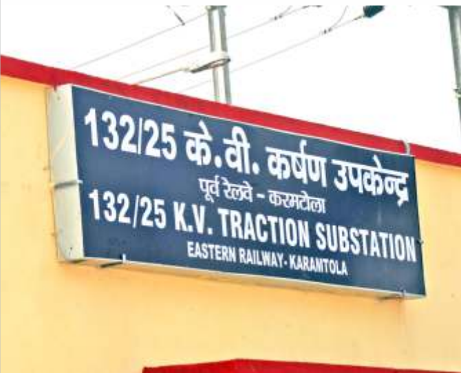
Electric sub-station at Karamtola
