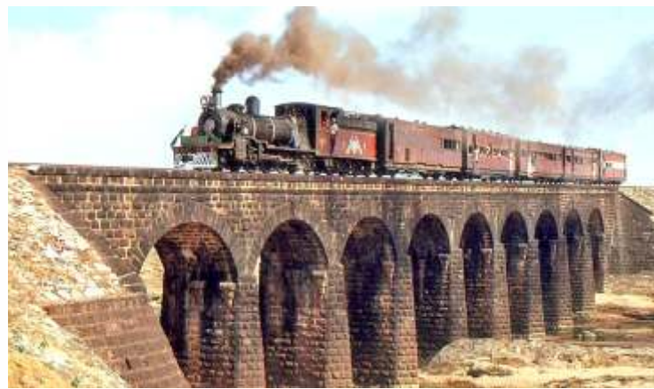
Another vintage Mayurbhanj train crossing an arch bridge
