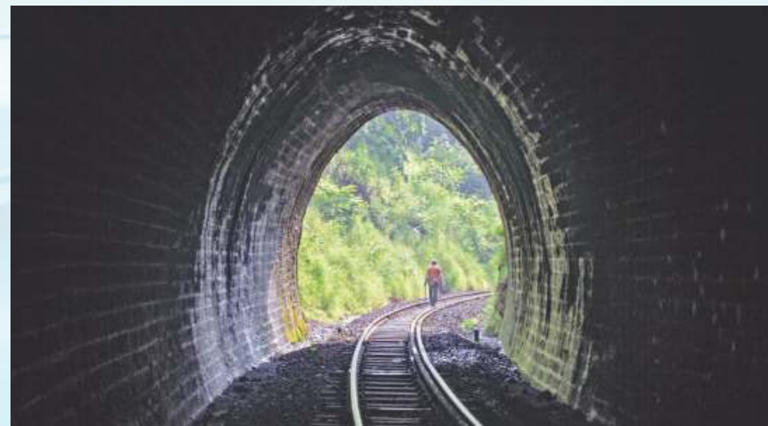
▲ Gangman inspecting track inside a tunnel
