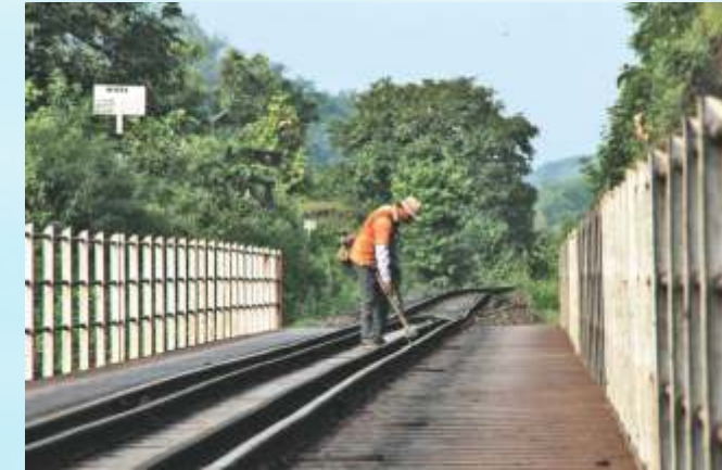
▲ A gangman inspects the line on Ravine viaduct No. 1
