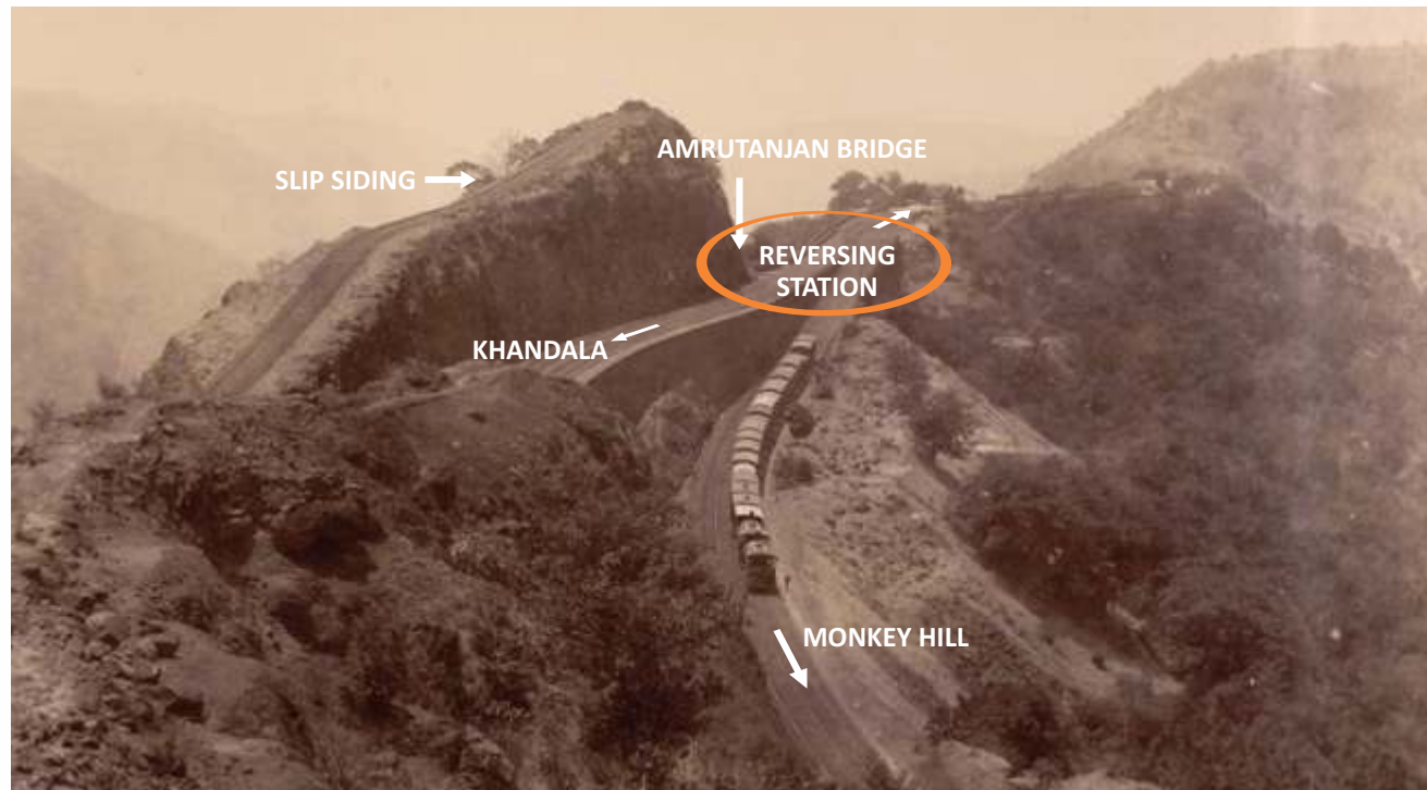
Fig.2 - Reversing Station - A view from top of Battery Hill
